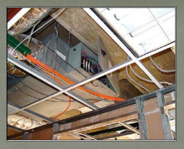
New provisions require access be provided for service and maintenance of electrical enclosures for resistance heating element type duct heaters which are mounted on a duct system. When installed above a ceiling the enclosure shall be accessible through a lay in ceiling or access panel.
