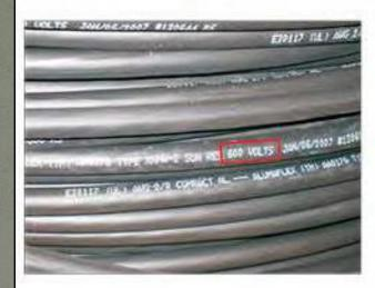
Numerous changes throughout the NEC from the 600 volts threshold to 1000 volts
