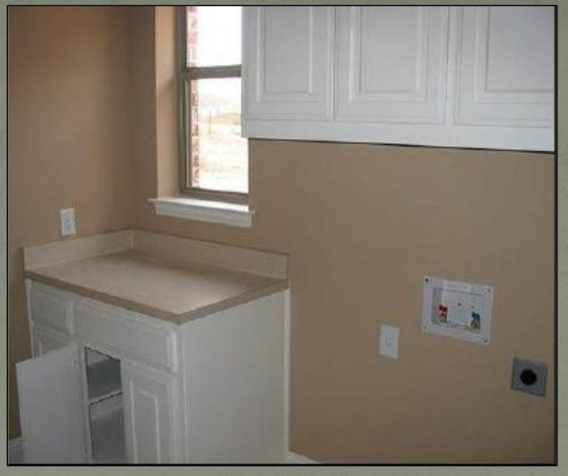
Now requires all 125-volt, single-phase, 15 and 20 ampere receptacles installed within a dwelling unit laundry area be GFCI protected whether a sink is installed or not.
