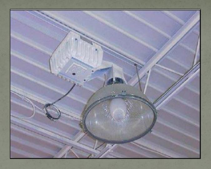
Luminaires are no longer allowed to be installed within 1½ inches of the lowest metal deck surface. This is to lessen the potential for roofing and decking fasteners damaging the luminaire or its wiring.
