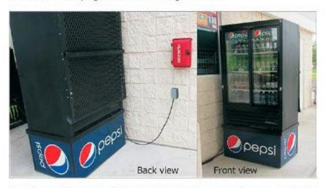
Vending machines not utilizing a cord-and-plug connection are required to be connected to a GFCI-protected circuit.
