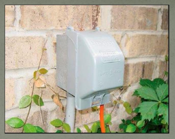
Extra duty covers are now required on all 15 and 20 ampere, 125 and 250 volt receptacles installed in wet locations. This includes dwelling unit wet location receptacles as well.
